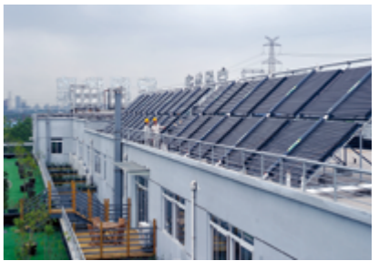
Rooftop solar water heaters of the logistic company of Baosteel Development
