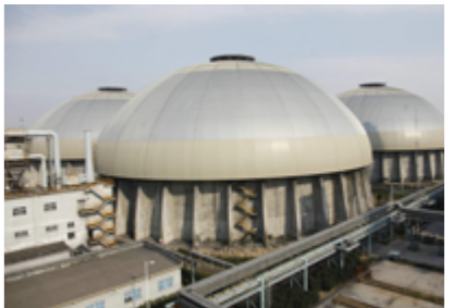
Closed raw material silo of Ningbo Steel
