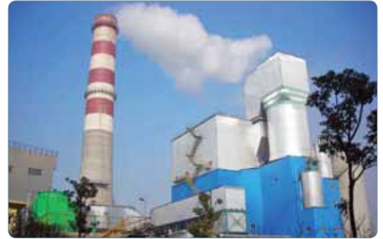
▲ The No. 4 sintering flue gas desulfurization unit of Meisteel employing the dry process - circulating fluidized bed was commissioned at the end of July 2009, with a desulfurization efficiency \geq 90\% and a 6,000 t/y reduction of \text{SO}_2 emissions.
