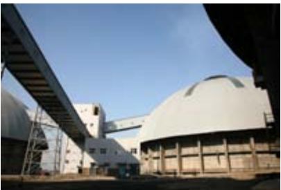
八一钢铁全封闭原料筒仓
