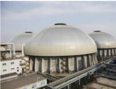
宁波钢铁全封闭原料筒仓
